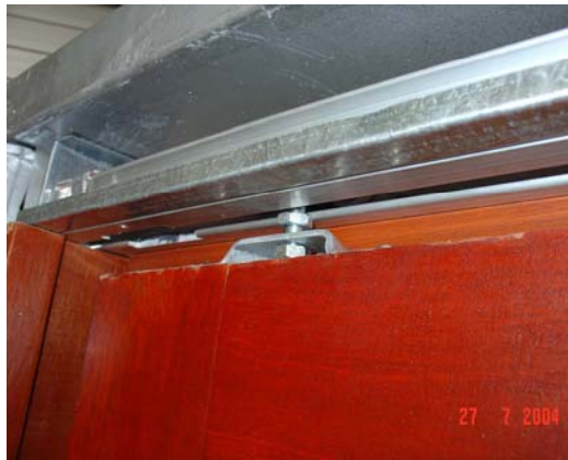
9. Hang door panel with the steel hanging bracket catching the Roller bolt
